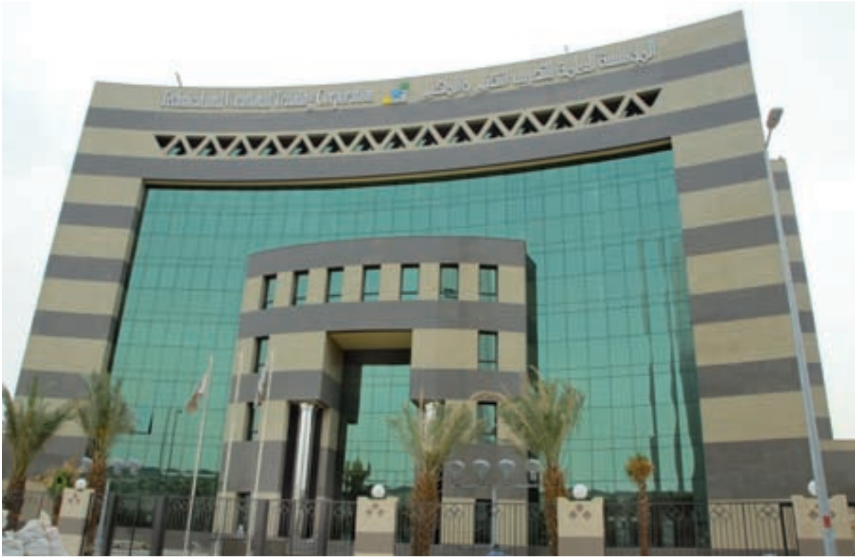
Gebäude der Technical and Vocational Training Corporation in Riad
